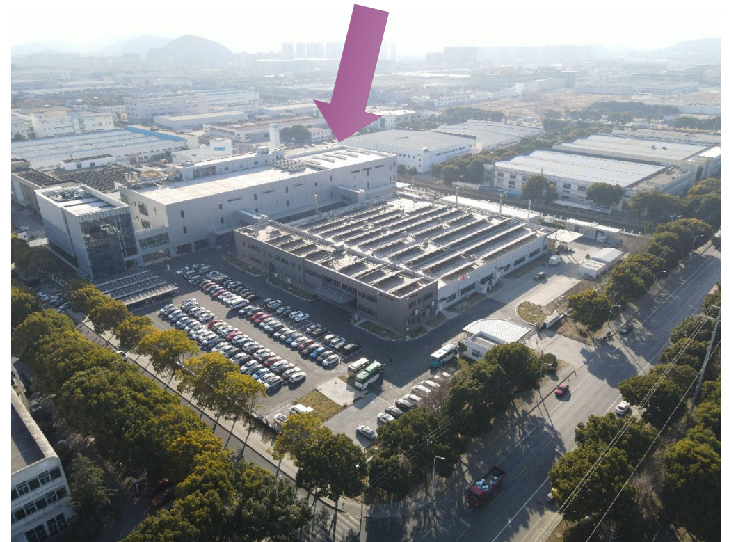
The expanded plant
